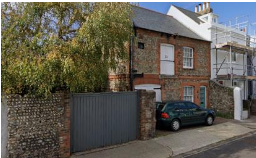
Figure 48: Park Road, west side
