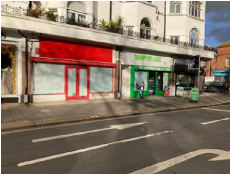
Figure 61: Poor quality shop fronts along Brighton Road
