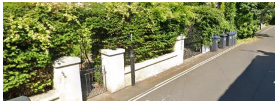
Figure 54: West side of Warwick Place
