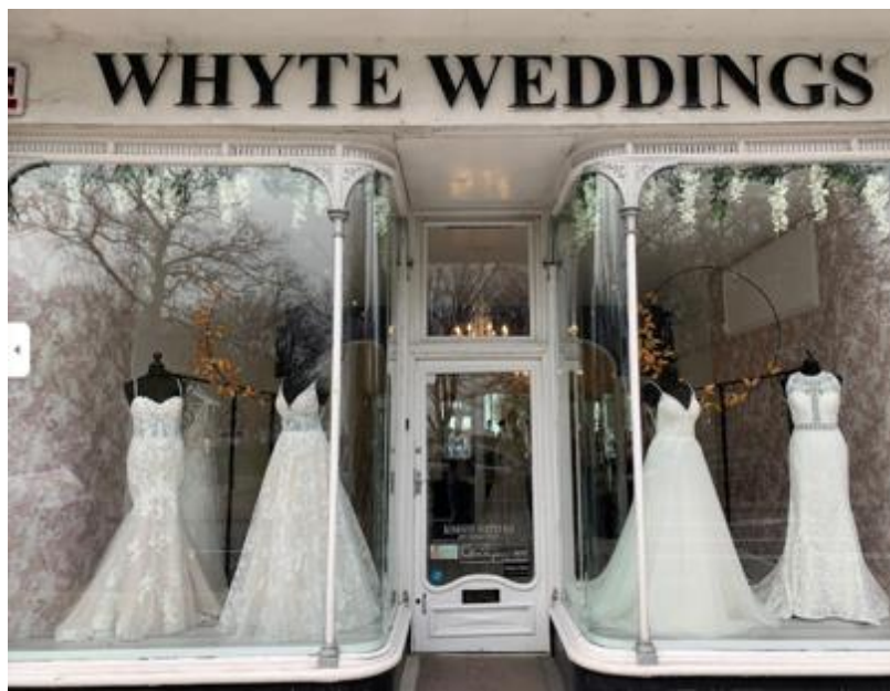
Figure 23: Shopfront at No.6 The Broadway
