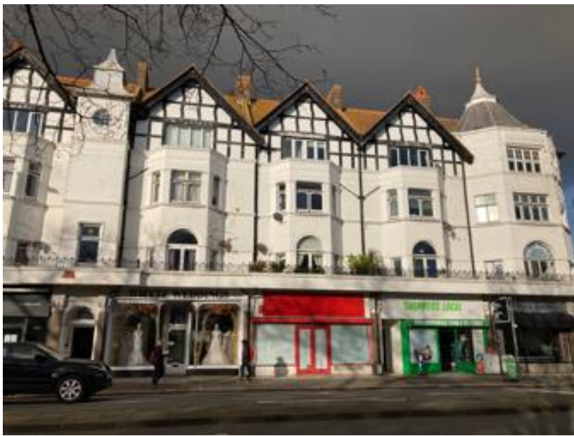
Figure 76: Variable quality shopfronts at Broadway Mansions
